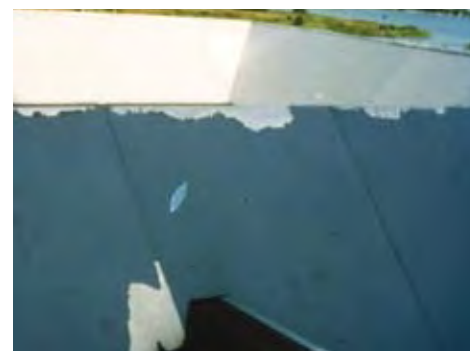
Img. 5.3.3. Blistering caused by cross-linkage
