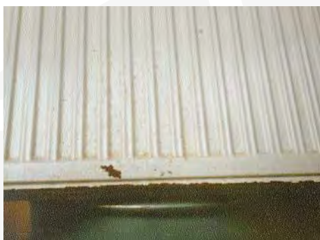
Img. 5.1.2. Infiltration caused by chemical exposure
