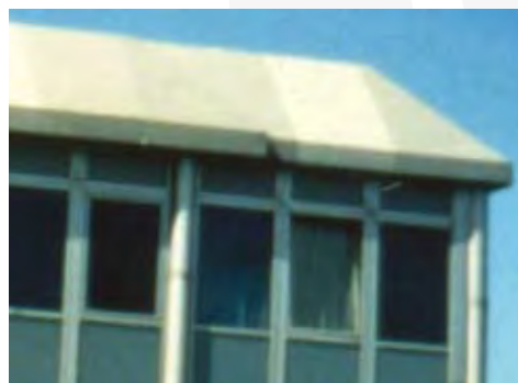
Img. 4.4.4. Color hue change caused by insufficient adhesion
