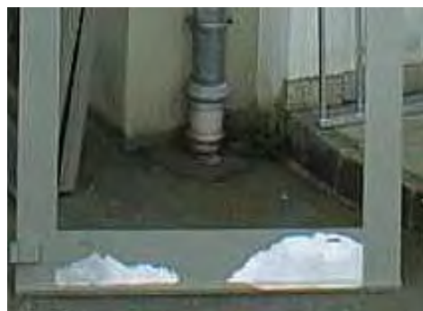
Img. 5.3.4. Blistering caused by an inappropriate pretreatment
